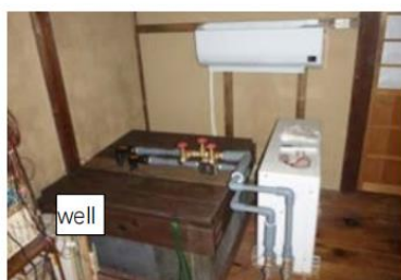
Fig. 3. Well and heat-pump system
