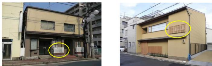
Figure 2. Blindfold fence for AC outer unit
